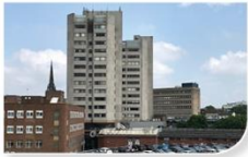
■ City Centre South Demolition of Coventry Point
