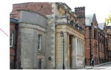
■ Drapers Hall - Drapers Hall - re-vamped
